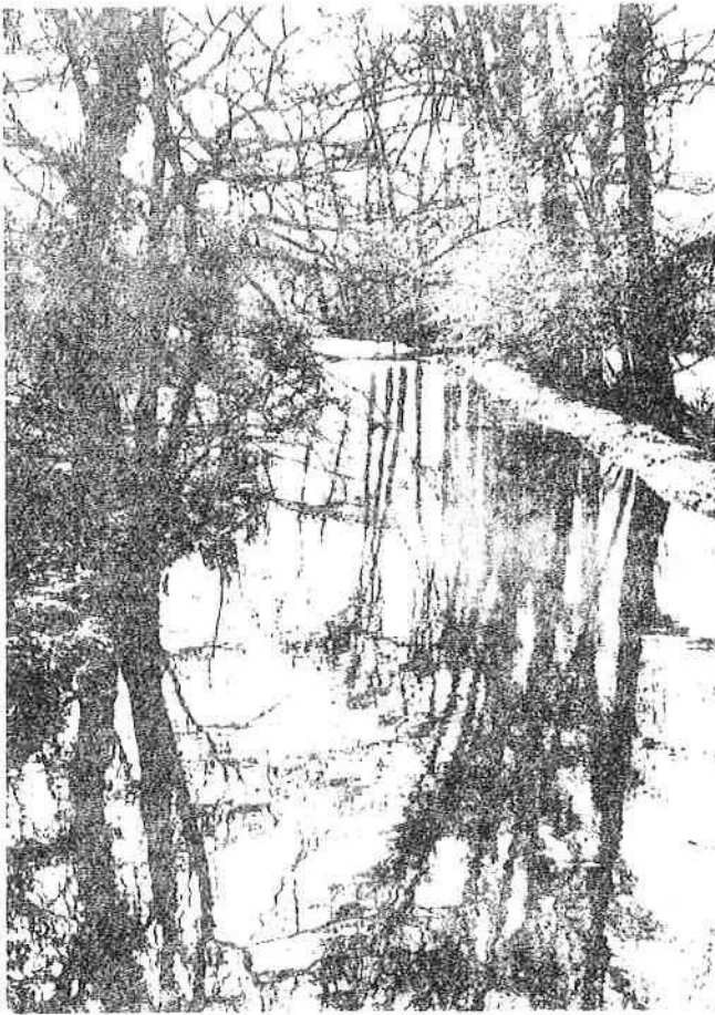
Plate 15.1 The Brownslover Arm feeder to the Oxford Canal (North) showing lack of bank protection. (PFP)
